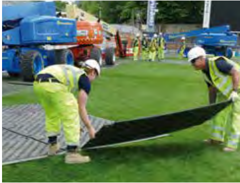
MaxiTrack mats quickly bolt together for rigid support.
